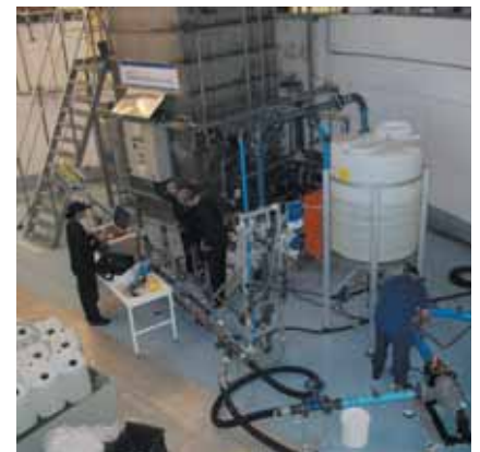
TEAMWORK: The CPUT team assembling the rig.
